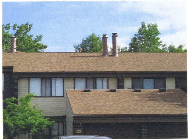
Asphalt shingle roof overview
