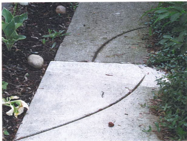
Diamond grinded section of concrete sidewalk
