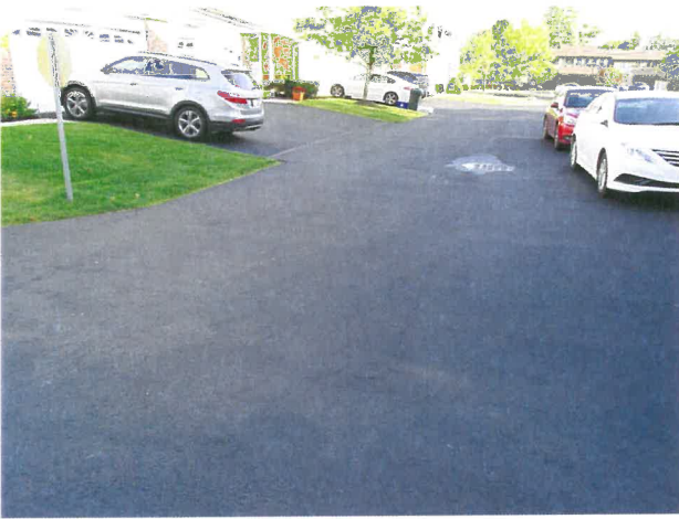
Asphalt pavement overview
