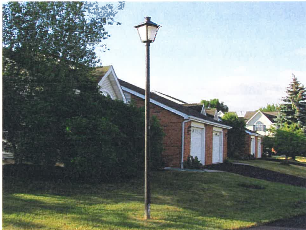
Light pole and fixture overview
