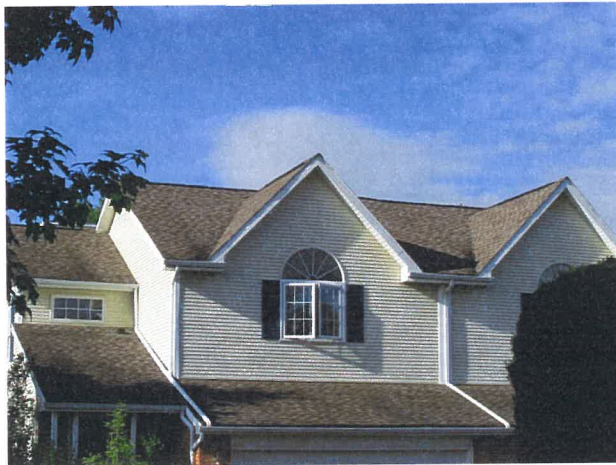
Asphalt shingle roof overview
