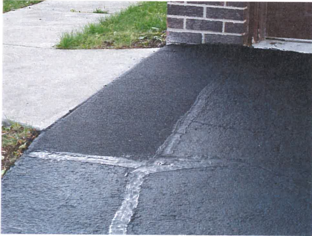
Pavement patch repair
