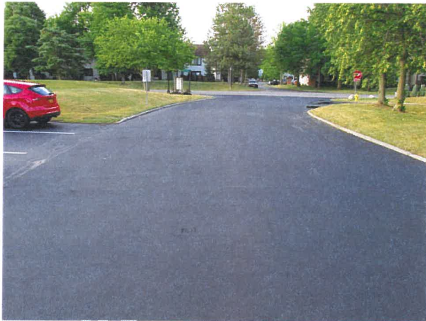
Asphalt pavement overview
