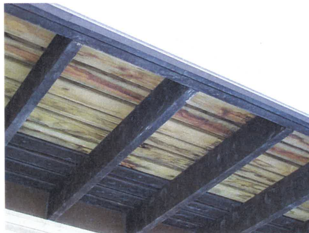
Partial replacement of balcony decking
